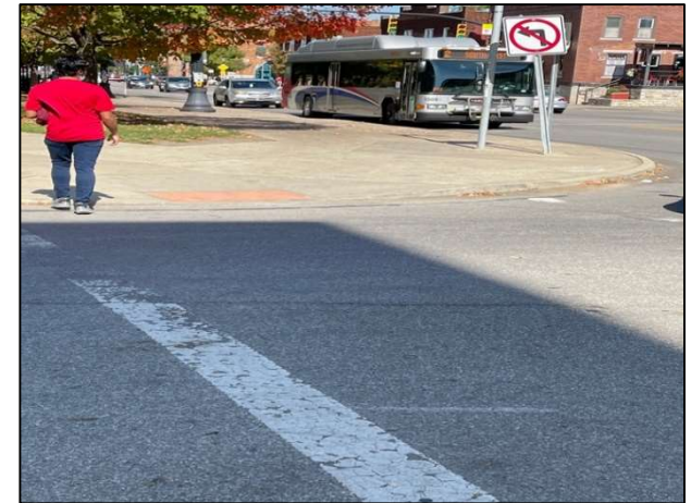
Poorly defined (no hash lines) and maintained crosswalk at 11 th and High Streets
