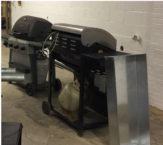
Liquid Propane Cylinders (LPG) stored inside of buildings
