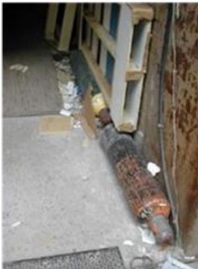
Compressed gas unsafe storage
